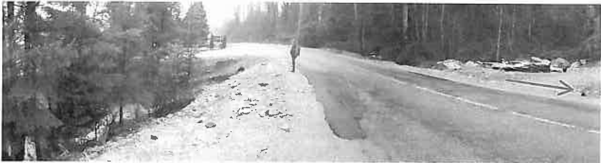
Photograph 37. Dale Creek downstream of the concrete culvert, which directs the creek below Sylvester Road. The cross-section at the point where the person is standing most likely will not contain the 200-year return period flood flow. The red dashed line delineates the area of the road fill that failed on October 17, 2003 due to culvert overtopping on the east side of Sylvester Road (shown by a red arrow on Photograph 36).
