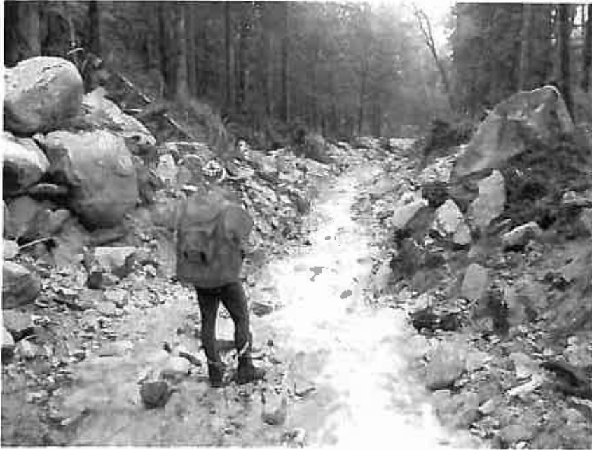
Photograph 30. Freshly excavated channel of McNab Creek 200 m upstream of Sylvester Road, December 8, 2003. The yellow lines show aggradation that was observed by BGC on Jan. 20, 2004.
