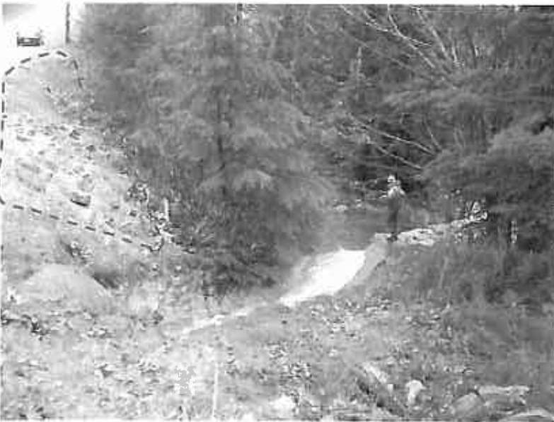
Photograph 37. Dale Creek downstream of the concrete culvert, which directs the creek below Sylvester Road. The cross-section at the point where the person is standing most likely will not contain the 200-year return period flood flow. The red dashed line delineates the area of the road fill that failed on October 17, 2003 due to culvert overtopping on the east side of Sylvester Road (shown by a red arrow on Photograph 36).
